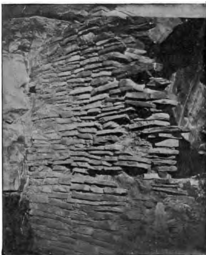
FIG. 250—Structure of wall of Honanki
